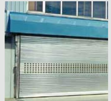
In case of internal lack of space, external rollers can be used. The weather-proof cladding can be architecturally appealing at the same time.
